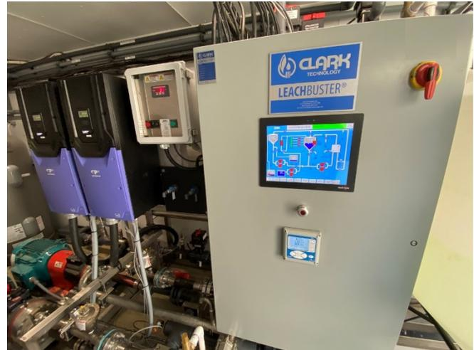
Photograph 2: Standard interior view of the control panel, pumps, VFDs, and other equipment for a typical Containerized WWTP. Virginia CLB is shown.
